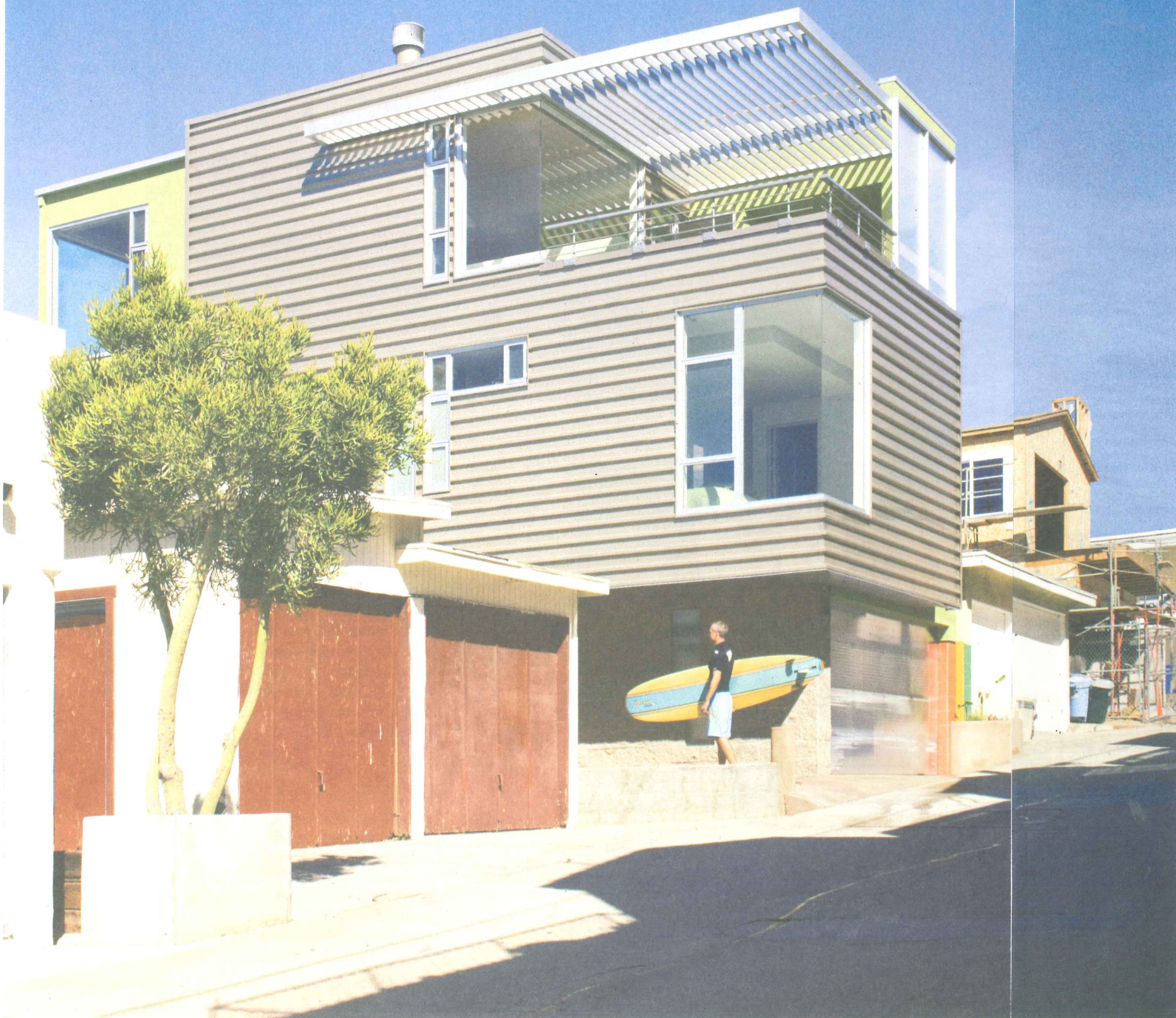
DAVID DUNCAN LIVINGSTON Sited on a back lot, the house is entered off an alley (opposite). The garage door is made of translucent polycarbonate. The steel cladding is extremely durable, low maintenance, and resistant to salt air. The skylight over the stair (above) opens automatically to vent the interior.
