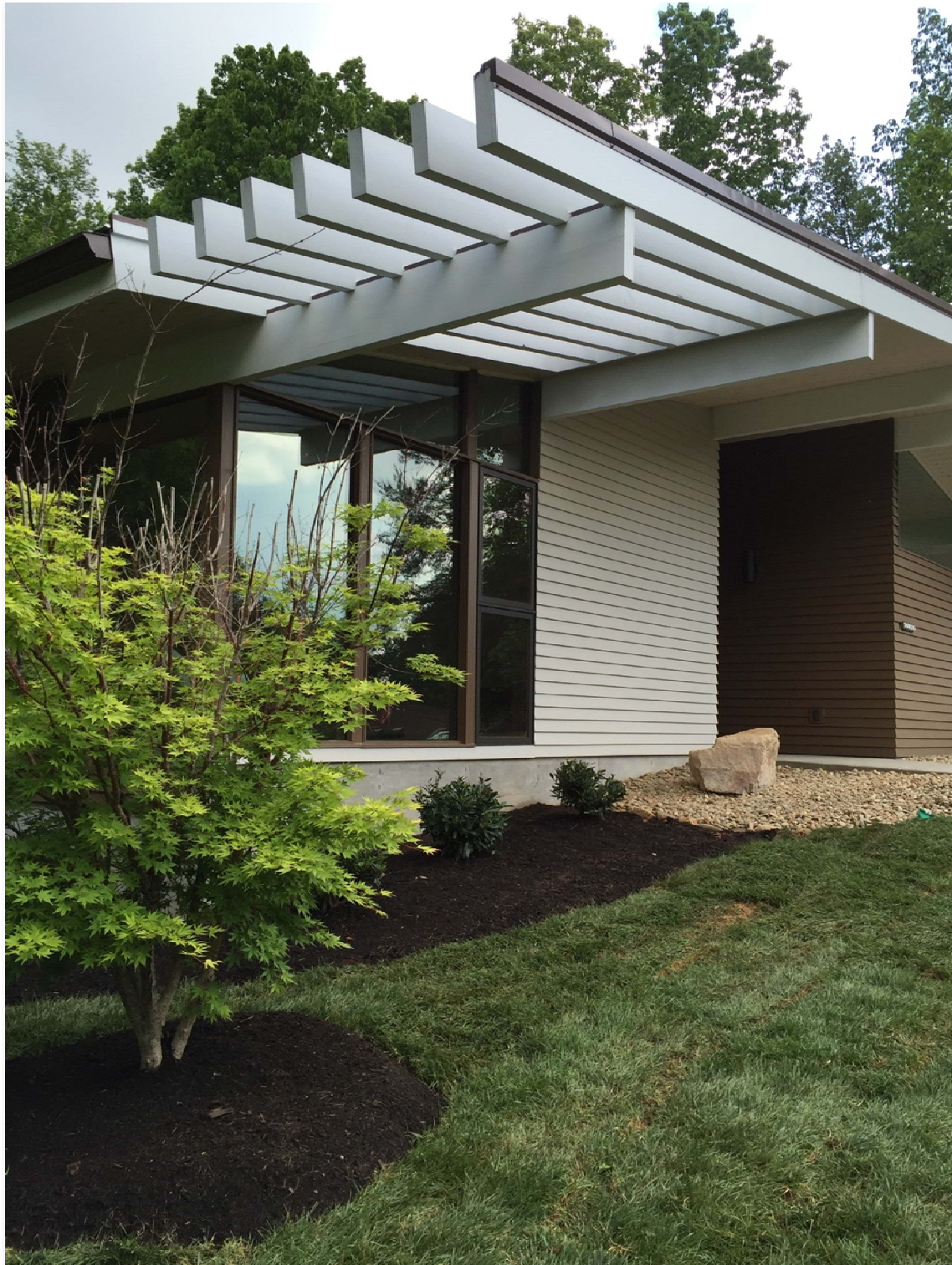
The trellis at front bedroom windows allow filtered light into the room. The cleft to the right leads to the front door.
