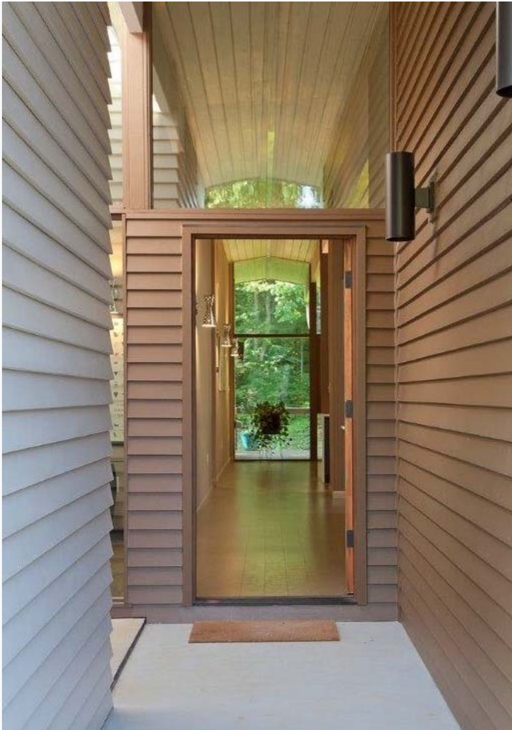
A skylight reveals the front door which, upon opening, immediately reveals the high glass window wall at the rear of the home....an architectural enfilade...
