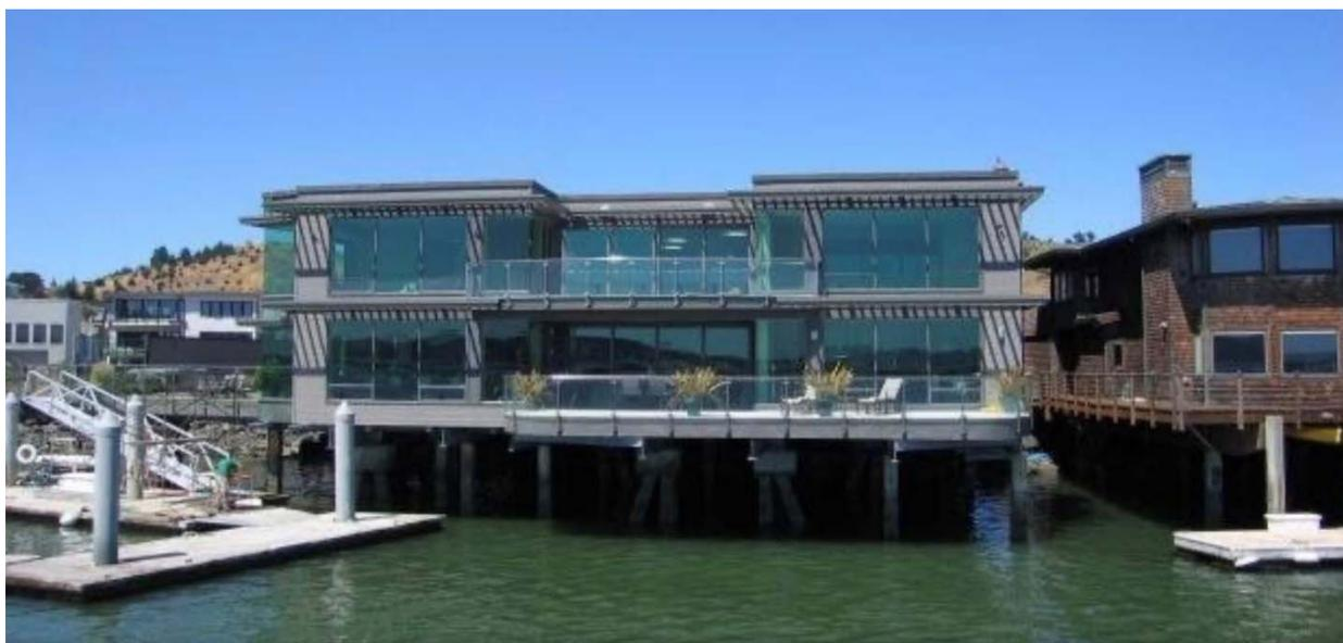
*The water side of the house has vast expanses of glass and decks. Powder-coated aluminum trellises provide solar protection as well as a computerized interior shade system*
