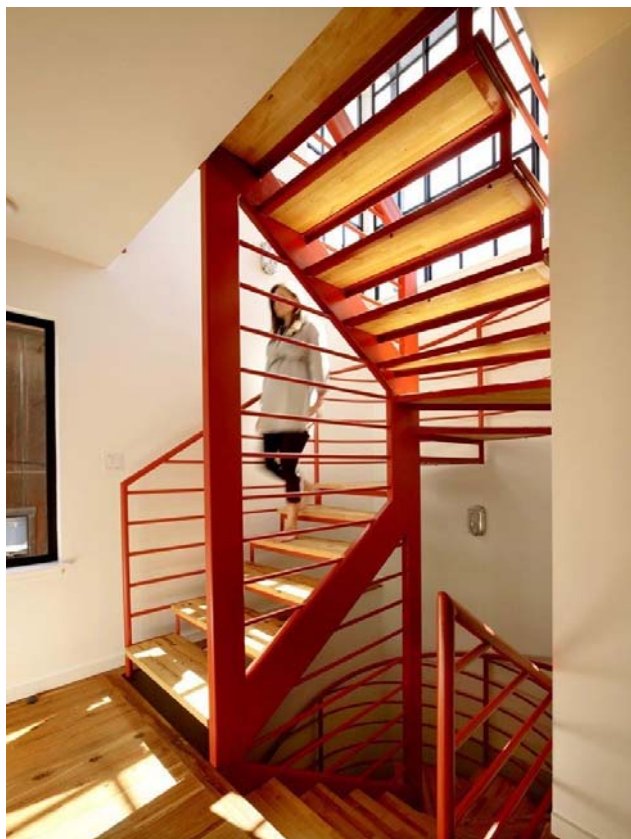
The free-standing metal stair services all three levels and is a method of bringing daylight to all levels. The stair has the same paint specifications as the nearby Golden Gate Bridge.
