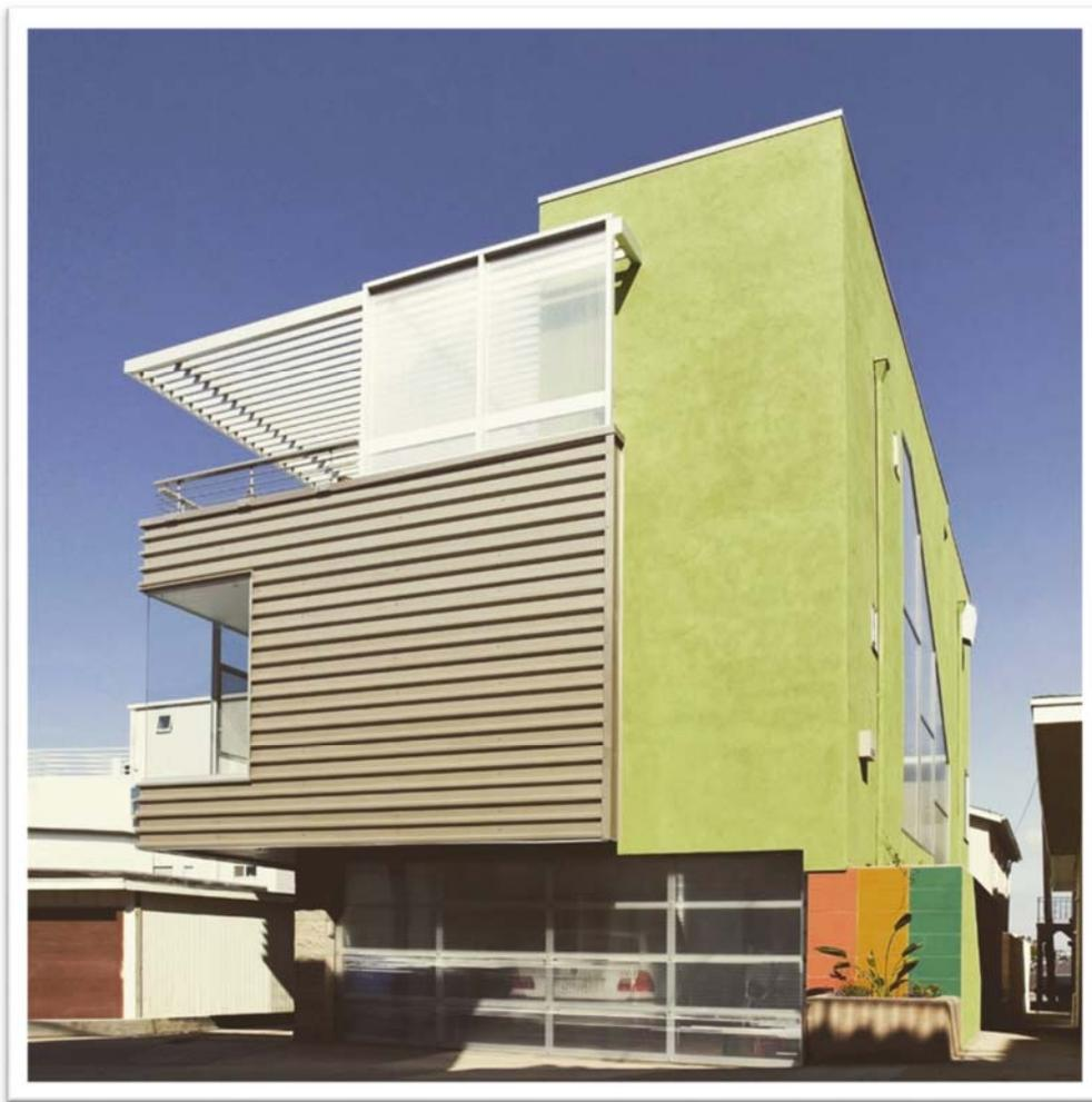
The exterior of the home is Avocado green elastomeric stucco and high-quality metallic silvery metal paneling, set horizontally as two durable exterior materials suitable for the coastline. Barbara says “The stucco installers were completely coated with green from head to toe and looked like aliens,” said Barbara. The silver metal panel system and the wall assembly it sheaths also shields the house from the intense summer and western sun.
