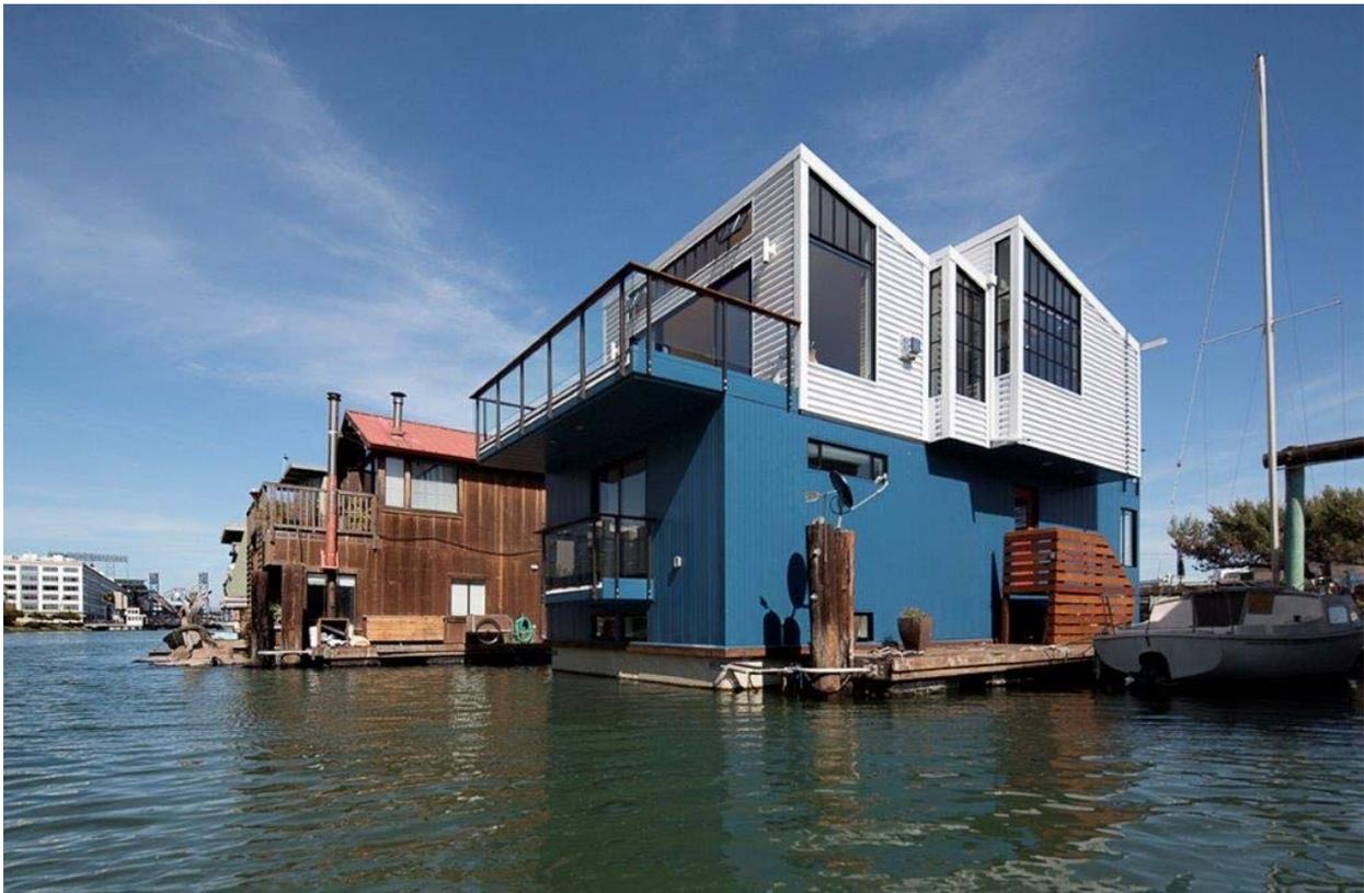
Marked by its sawtooth roof and shipping container-like facade, the home is moored to the dock alongside boats. Since there's no way to paint a floating house, Nebolon chose to clad the exterior in 24-gauge metal siding coated with a fluorocarbon finish that will resist fading and chalking for 40 years. "It's a very durable paint system that doesn't require periodic painting," he explains. "An annual hose-down will work just fine."
